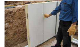
installing the insulated panels
