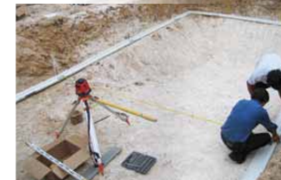
check levels and construct pool
