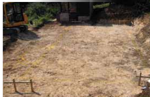
clear site and marking out
