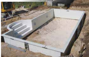
pool structure built
