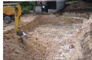
excavation as per drawing
