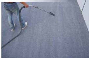
clean site and vacuum underfelt
