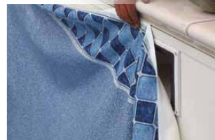
apply the liner
